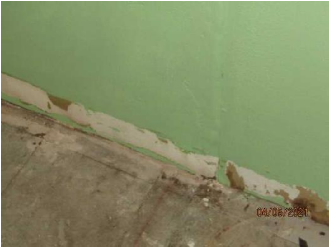
Dwelling/Interior/Basement Bathroom - 23-IMG_0023
