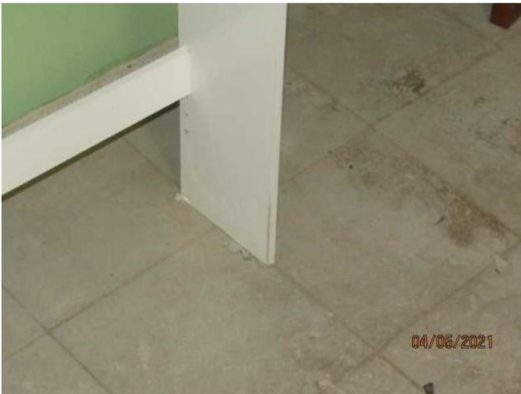
Dwelling/Interior/Basement Bathroom - 15-IMG_0015
