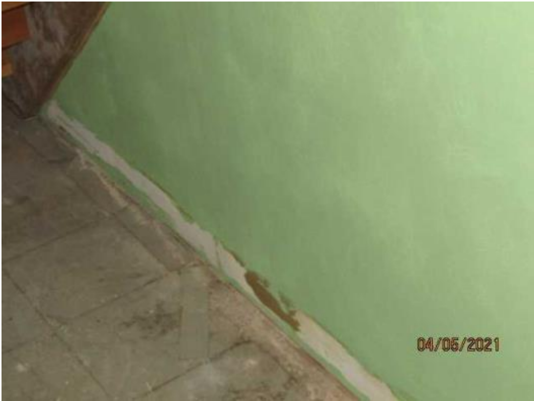
Dwelling/Interior/Basement Bathroom - 22-IMG_0022
