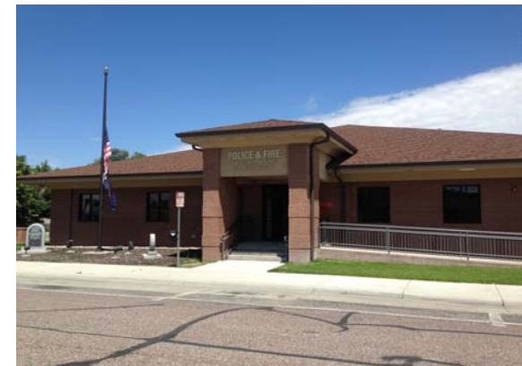
Public Safety Building - West 18th & Avenue B
