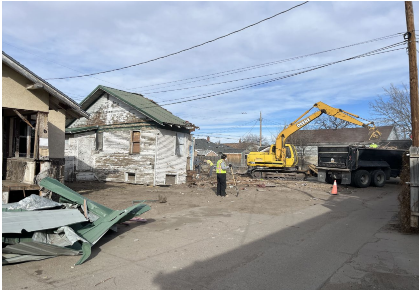
Demolition of uninhabitable homes
