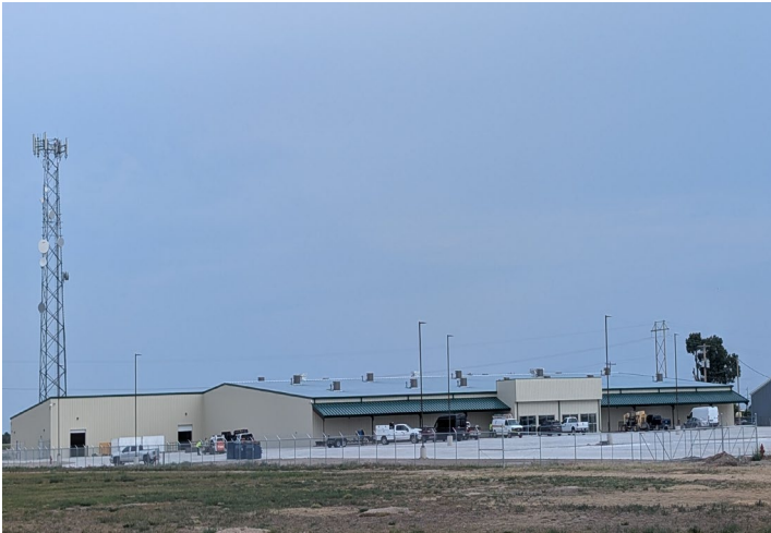
New Boomgears building
