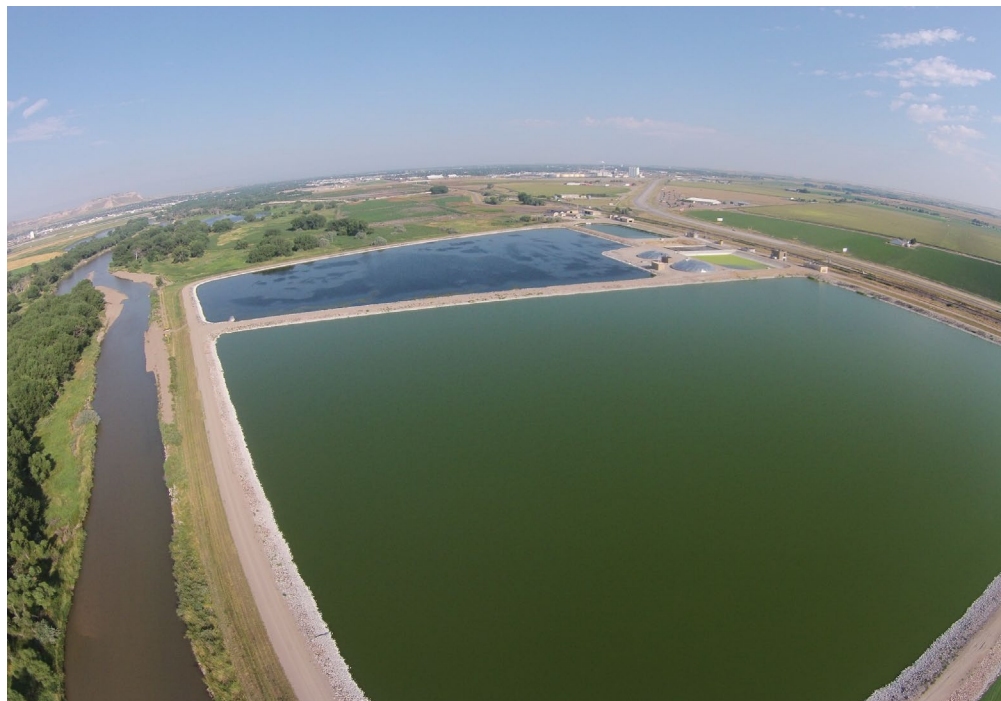
City of Scottsbluff, Wastewater Treatment Plant
