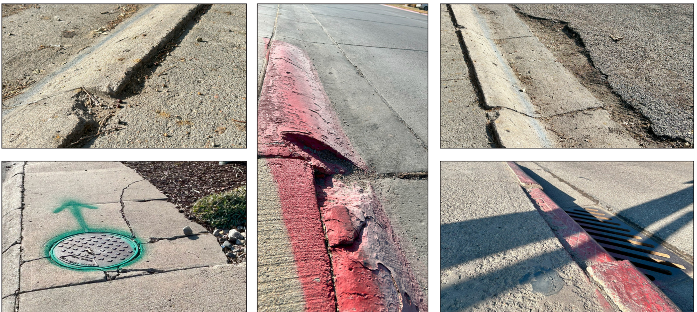
Examples of Curb, Gutter, Sidewalk Conditions within the Study Area
